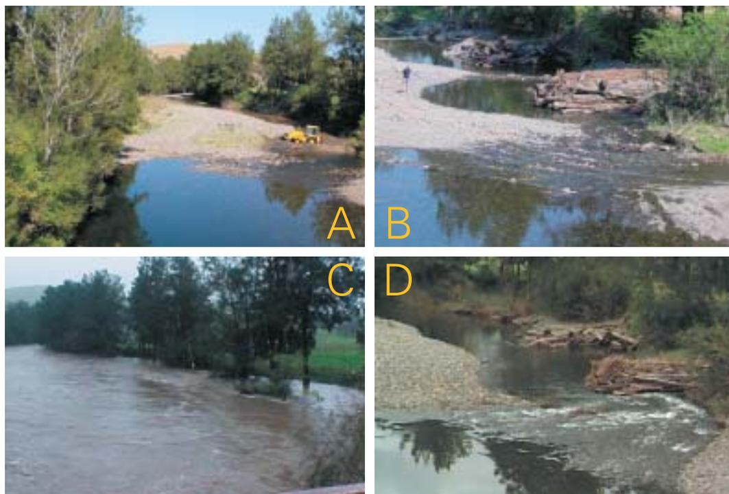
**These photos (A–D) show the construction of an engineered log jam that is designed to increase aquatic habitat and diversity in the river channel. Even after the large flood shown in Photo C the log jam remained in place, with Photo D showing how the log jam structure is changing the river channel to create a range of different habitats for plants and animals. Williams River, NSW.** Photos Andrew Brooks.
