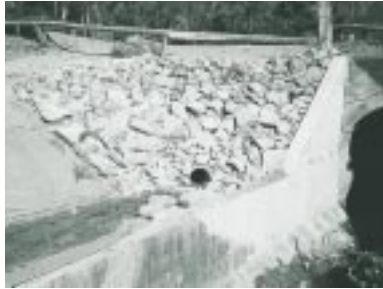
Low flow diversion pipe and overflow channel
