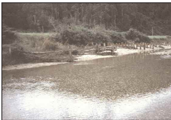
Figure 15. Pin retards and brush retards used to stop bank erosion and stabilise an artificial bench on Taylors Arm, a tributary of the Nambucca River, in northern New South Wales.
