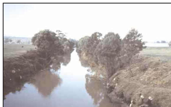
Figure 39. Twenty kilometres of the Moe River in Victoria has been straightened and original meander bends have been backfilled, making reinstatement of meander cut-offs uneconomical.
