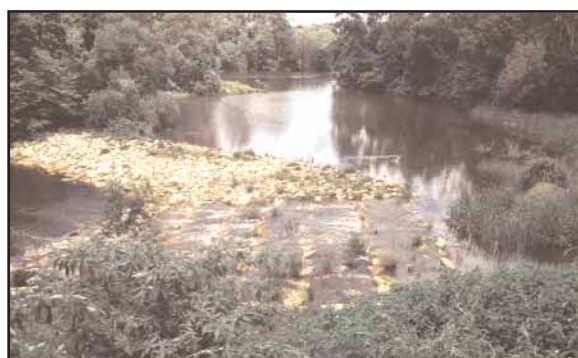
Figure 46. A zigzag fishway, with transverse ridges of rock that effectively reduce the slope of the fishway (photo by John Harris).
