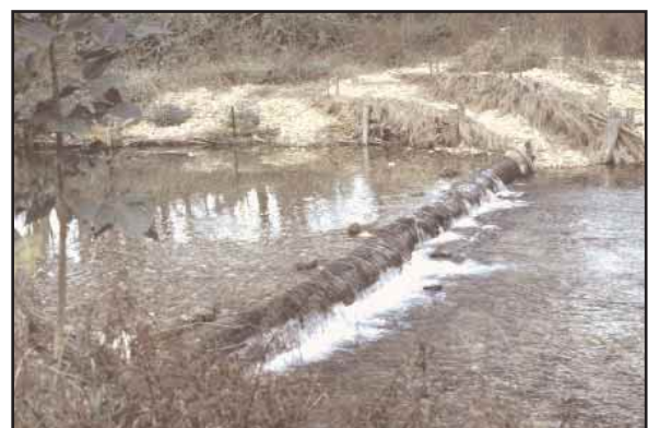
Figure 9. A flat-crested log dam on Taylors Arm, a tributary of the Nambucca River in New South Wales (photo by Allan Raine).
