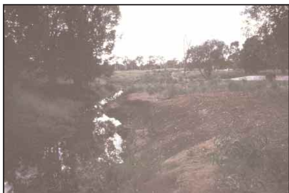
Figure 26. Camphor laurel mulch held down with geotextile webbing while replanted revegetation is establishing on the banks of Kelly's Creek in Brisbane.
