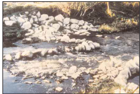
Figure 13. An example of a Mangfall sill with a central fishway (photo by Wal Hader).
