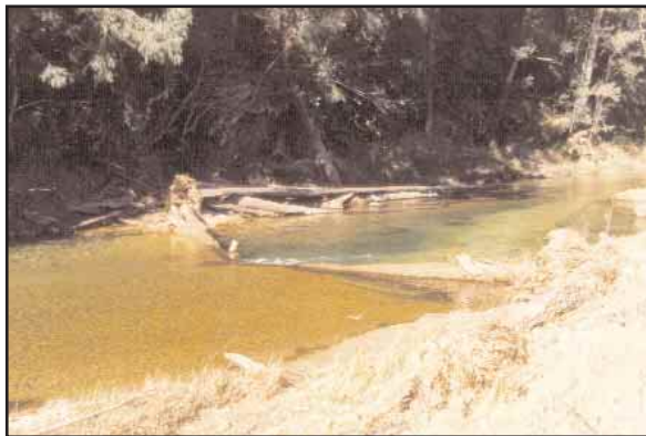
Figure 12. A Schauberger sill (flow from left to right). Note that the apex of the sill is the lowest point, and is pointing upstream. As a result, the flow is concentrated in the centre of the channel, and there is a deep scour pool downstream of the structure (photo by Wal Hader).
