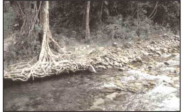
Figure 63. Undercutting of the bank in Babinda Creek in far north Queensland.
