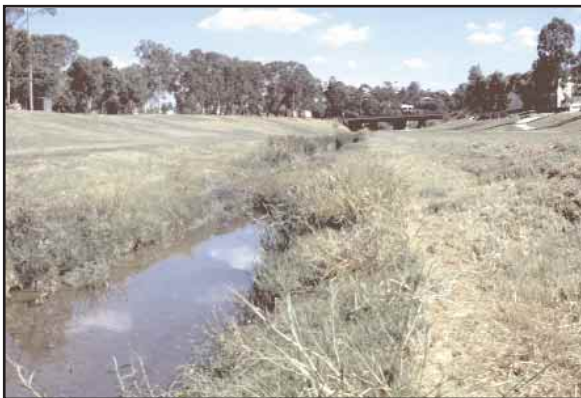
Figure 23. To achieve maximum flow conveyance, many streams have been cleared and straightened, as in this example of Downfall Creek in Brisbane.
